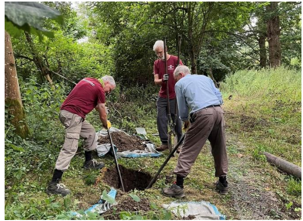
Preparing holes for deer-proof fencing
